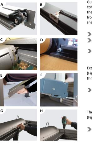
Guide the pull belt inside the guide rails f**rom below** over the lower connecting roller back to the front profile (Fig. A) and place the eyelet over the pull hook (Fig. B). Push the pull hook into the intended channel on the front profile to the stop (Fig. C), the snap fastener here makes a clear snapping sound. The pull belt tension should be approx 200 mm - 600 mm.
