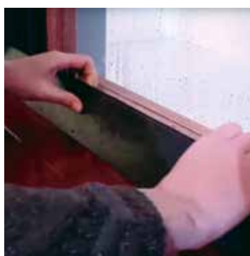
The cover profile is easily clicked open.
